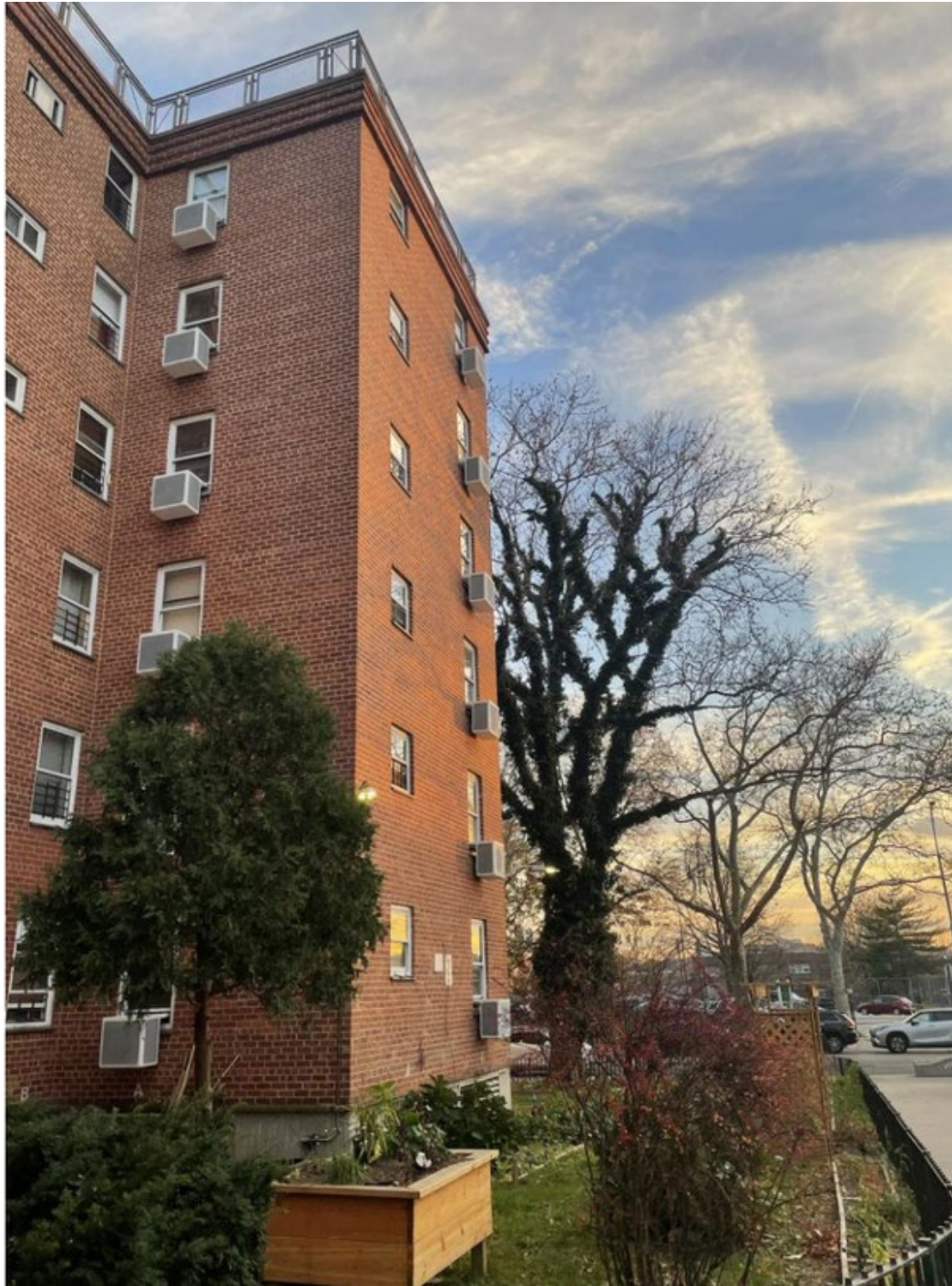
Exterior View of the Midea units at Woodside Houses
